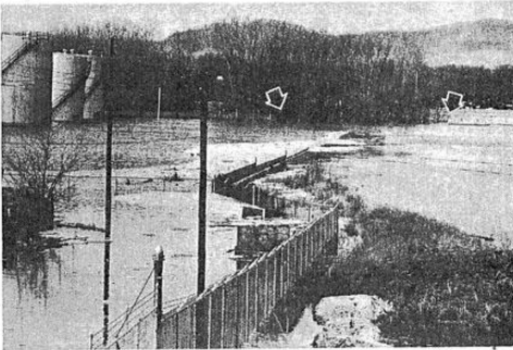
ARROWS INDICATE AREA WHERE DIKE BROKE MONDAY Center Oil Storage Tank Has Tipped Slightly.
