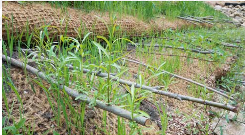
Live stakes will grow new shrubs at the restored Lyndale Avenue outfall
