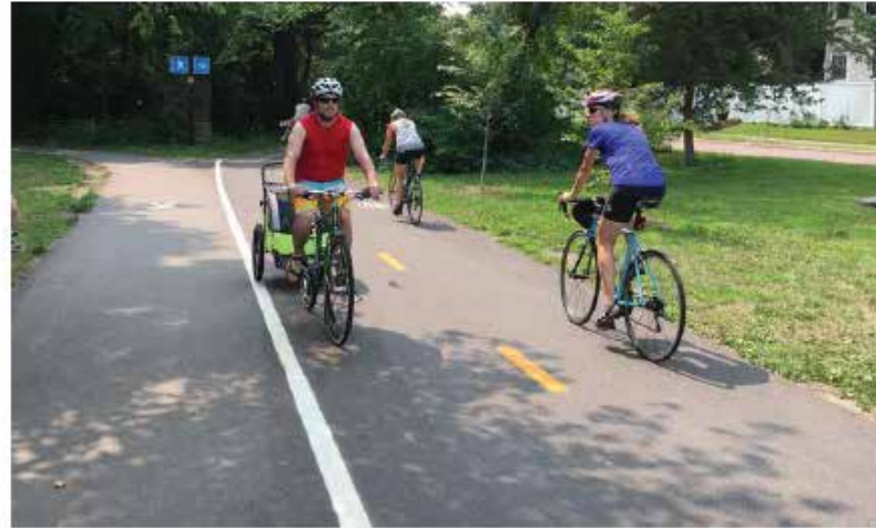
Typical mode-separated off-street trails along Minnehaha Parkway Regional Trail
